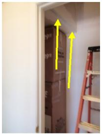
The drywall in the small walk in closet is not completed
