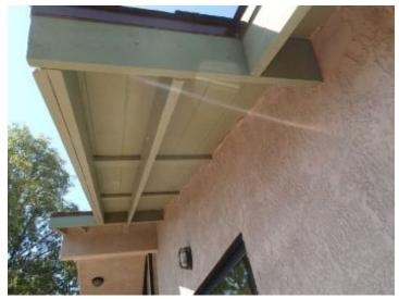
Visible eaves appear to be in good condition with Visible eaves appear to be in good condition with normal wear and weathering. normal wear and weathering.
