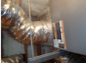
The air ducts were visually inspected and found to be in good shape and tightly connected to the plenums and register boots.
