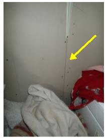
The wall between the living area and the garage is The wall between the living area and the garage is a fire wall with a unprotected opening.
