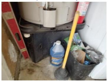
When the water heater leaks it will be onto the floor. Any items stored on the floor will be subject to water damage.
