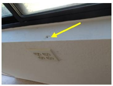
There are small holes in the wall that will need to be filled and painted by the window sill, center
