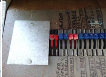
The electrical service is a 100 amp meter main was visually inspected and found to comply with has no evidence of burning or arcing.
