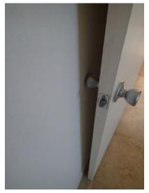
Door stop missing allowing the knob to damage the wall.
