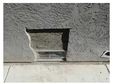
The stucco over the vent screen at the side of the yard has not been completed
