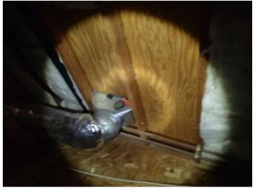
There is a small section of the attic wall by the kitchen that is missing insulation
