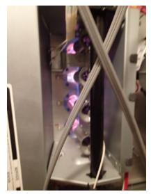
The heating unit is a natural gas fed, horizontal forced air unit. It was visually inspected and then placed into the heating mode. The unit functioned as designed.
