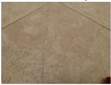
The stone has a hairline fracture running from left to right across the floor
