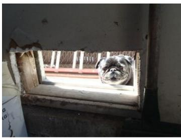
The screening over the vents grill is torn or missing and no longer an effective stop for rodents or insects at th front of the garage
