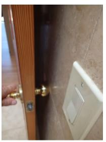
The door stop is not installed allowing the door knob to strike the wall in this area
