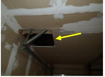
The ceiling in this area is a fire rated ceiling and is The ceiling in this area is a fire rated ceiling and is not allowed to have unprotected openings such as areas cut out.
