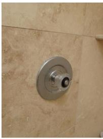
Hot and cold reversed with the hot at the full clockwise position. This is a scalding hazard
