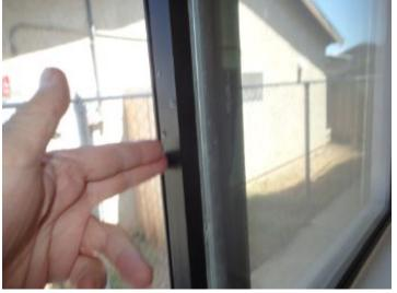
The window latch/lock hardware is missing
