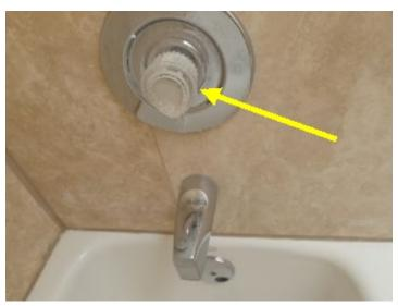
The valve no longer has positive stop at full hot or cold but rotates through 360 dgs.
