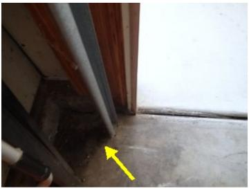
This door is not equipped with a safety-eye beam used to detect the presence of kids or animals running under the door while it is closing.
