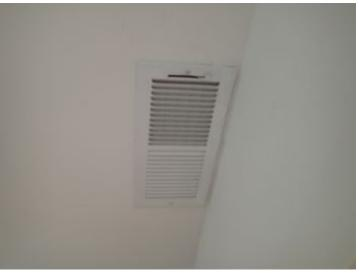
FYI: closing the registers in unused spaces might feel like you are conserving energy. In reality, this raises the air pressure of the system, making the fan work harder and reduces total air flow at the heater which limits the amount of heat captured from the gas. This usually results in a net energy loss. The register covers are best to be left at least partially open
