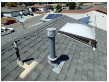
Correctly installed flashing with correct shingl lap on the back side
