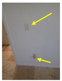
The 1/2 hot wall switched outlet is located below the wall switch
