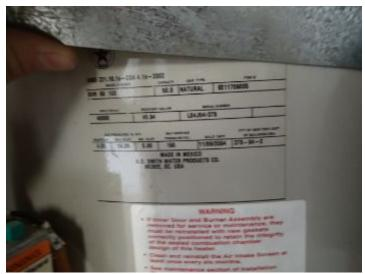
Functional, the tank was manufactured in 2004 . Typical expected life of a water heater is 10 to 15 years.
