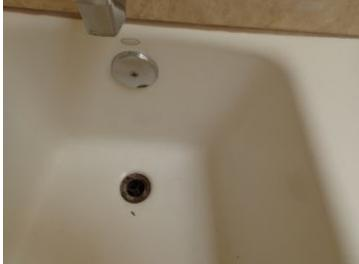
The tub stopper is missing making this functionally a shower only
