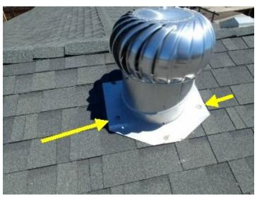
There are 3 roof jacks on the front side that are installed without the shingles running over the uphill portion of the jack down to at least the center line of the pipe
