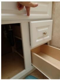
The cabinet top drawer will not close completely because it hits the water line at the back
