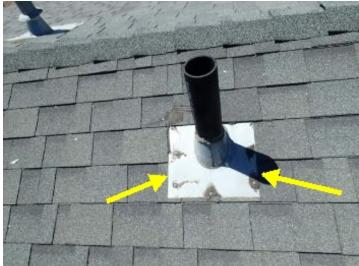
There are 3 roof jacks on the front side that are installed without the shingles running over the uphill portion of the jack down to at least the center line of the pipe
