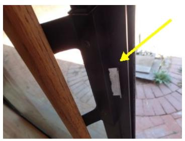
The sliding door lock does not unlock properly, it needs repair or replacement
