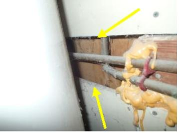
The wall between the living area and the garage is a fire wall with a unprotected opening.
