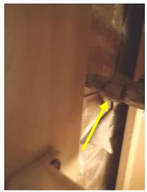
The cabinet top drawer will not close completely because it hits the water line at the back
