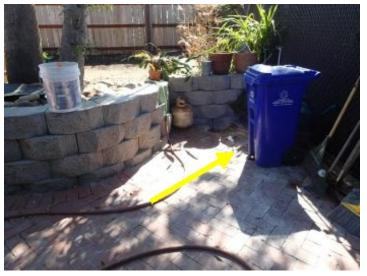
The patio is concrete which is in good condition in The patio is not complete in the rear right corner the front with a minor shrinkage crack
