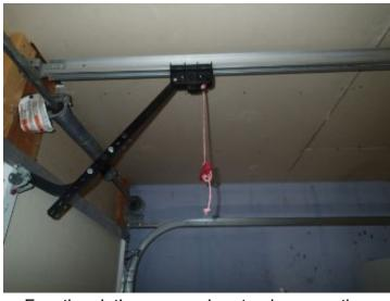
Functional, the garage door tracks, mounting hardware, springs and points of attachment were all inspected and found to be in good condition.
