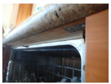
The dishwasher unit is securely fastened in place and attached to the cabinet top
