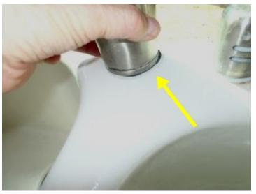
The faucet is not set tight to the deck. The faucet needs to be tightly fastened to and sealed to the deck to prevent water intrusion into the cabinet below
