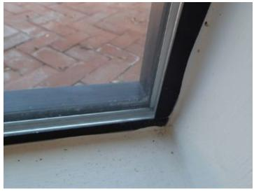
The window bottom is closer the 18" to the floor and is safety glass
