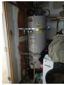
The water heater is on a platform in the garage in a location free from or protected from vehicle damage
