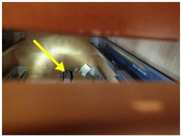
Outlet covers missing which could lead to accidental contact with live electrical parts. Located in the cabinet for the garbage disposer and on both side of the island cabinet
