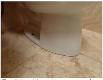
The toilet bowel does not have a waterproof seal at the junction of the floor. This creates a concealed fouling for moisture and organic groweth.
