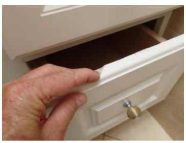
There is finish is degraded on the front of the cabinet drawer front top edge
