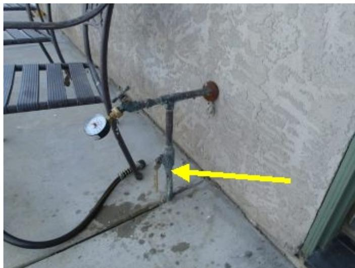
The building water shut off is located on the front of the house to the left of the front door.
