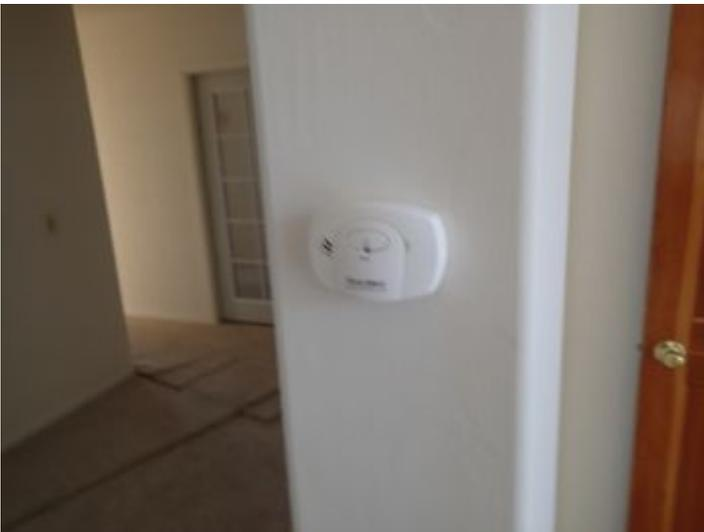
Carbon monoxide detector is in place on the hall wall
