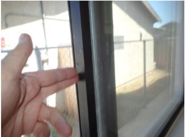
The window latch/lock hardware is missing
