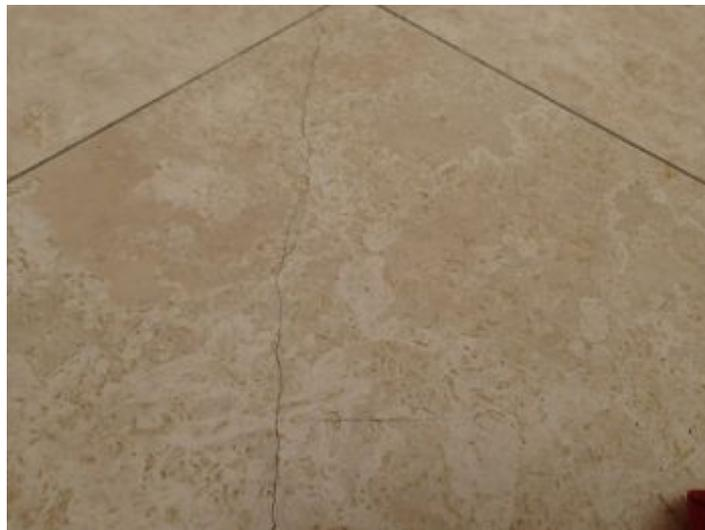
The stone has a hairline fracture running from left to right across the floor
