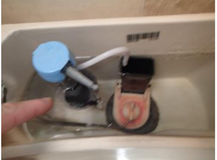
The fluid master flush valve did not shut the fill water off, it needs repair or replacement
