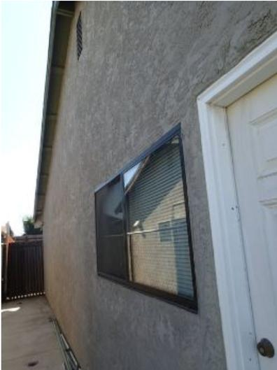
Stucco is in sound condition with no major cracks or holes present
