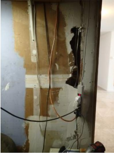
The wall between the living area and the garage is a fire wall with a unprotected opening.
