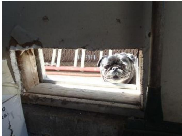
The screening over the vents grill is torn or missing and no longer an effective stop for rodents or insects at th front of the garage
