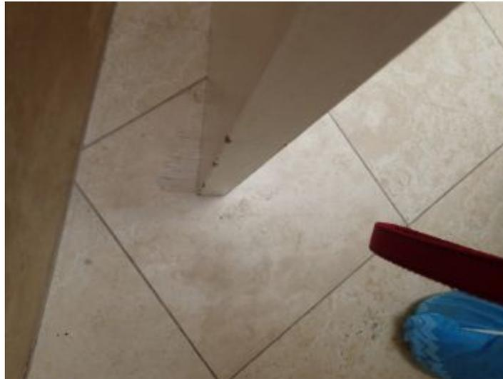
The door bottom drags on the floor when almost completely open and has scratched the floor
