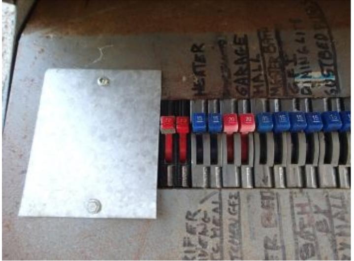
The electrical service is a 100 amp meter main with distribution. It is underground feed. The panel was visually inspected and found to comply with current safety standards. The interior of the panel has no evidence of burning or arcing.
