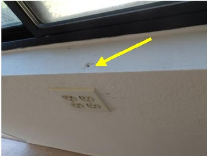
There are small holes in the wall that will need to be filled and painted by the window sill, center
