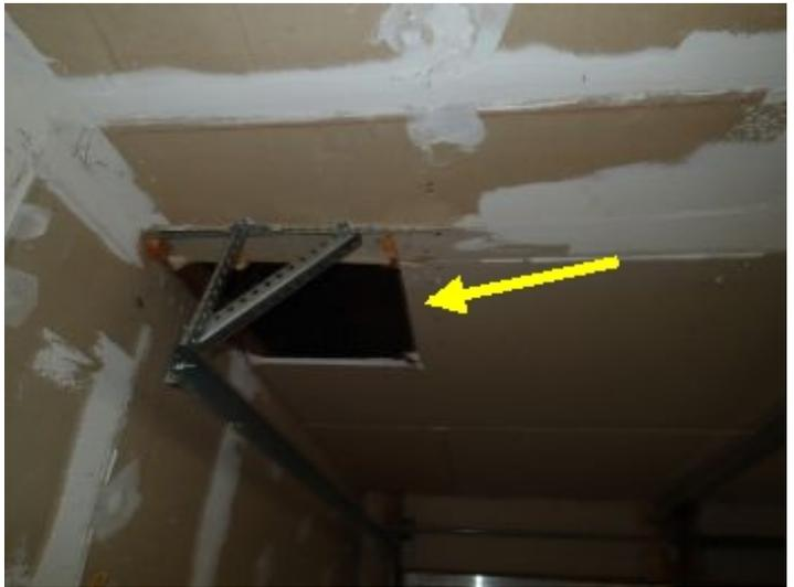
The ceiling in this area is a fire rated ceiling and is not allowed to have unprotected openings such as areas cut out.
