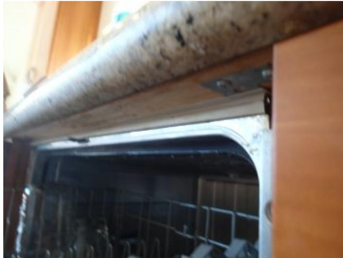
The dishwasher unit is securely fastened in place and attached to the cabinet top
