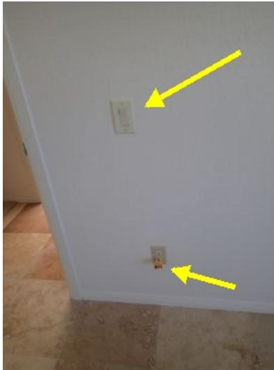
The 1/2 hot wall switched outlet is located below the wall switch
