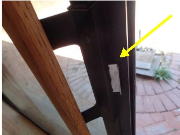
The sliding door lock does not unlock properly, it needs repair or replacement
