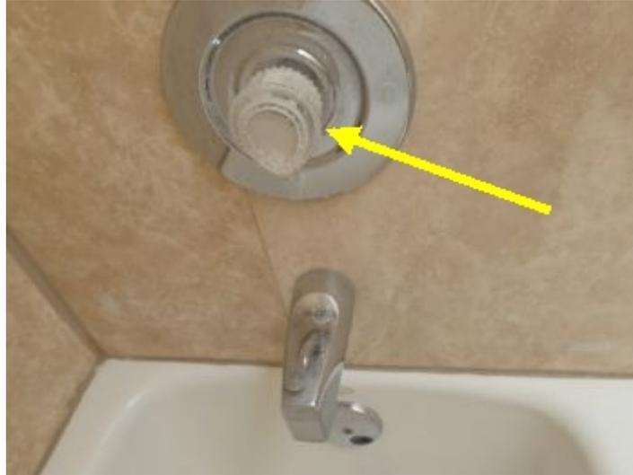
The valve no longer has positive stop at full hot or cold but rotates through 360 dgs.
