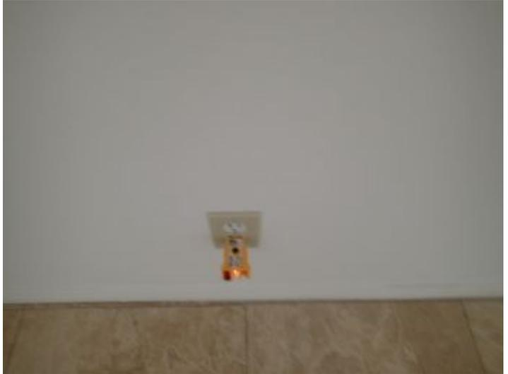
There are 3 prong grounding receptacles installed that do not have a ground connection. This is the outlet on the wall common to the hall bath
