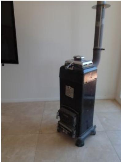
There is a wood or coal burning stove in place in the family room. It is an older unit, without any UL rating or installation requirement minimum to inspect to. Recommend that this installation be reviewed by a fireplace/wood burning stove specialist
