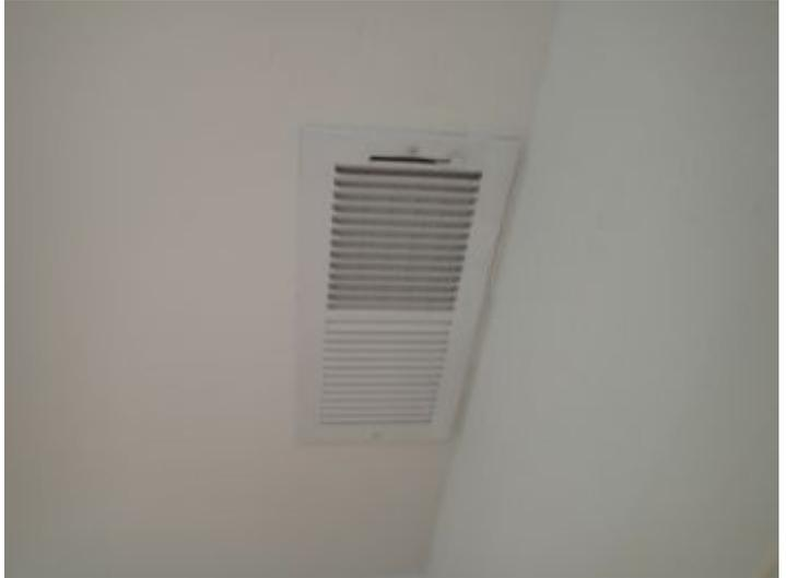
FYI: closing the registers in unused spaces might feel like you are conserving energy. In reality, this raises the air pressure of the system, making the fan work harder and reduces total air flow at the heater which limits the amount of heat captured from the gas. This usually results in a net energy loss. The register covers are best to be left at least partially open
