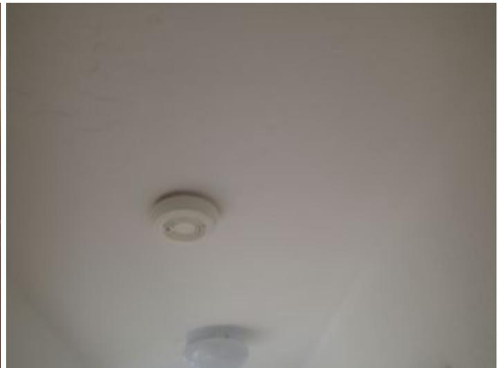
The required smoke detector is on the ceiling in the hall
