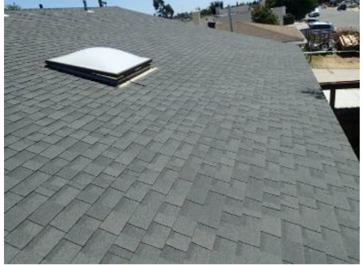
The roofing materials has good granulation retention. The shingles are laying flat and firmly attached. No signs of wind damage or missing shingles
