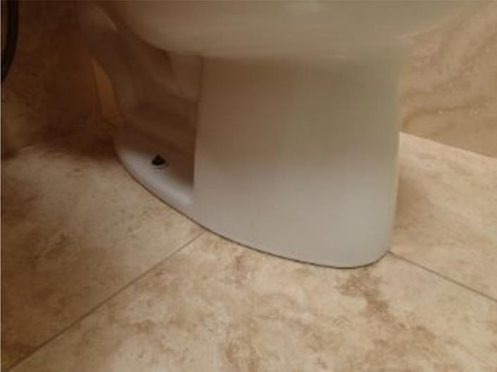
The toilet bowl does not have a waterproof seal at the junction of the floor. This creates a concealed fouling for moisture and organic growth.
