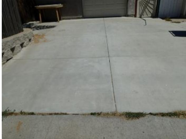
The driveway and walkway are in good condition with no significant settling or cracking.
