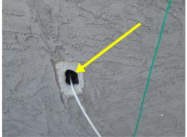
The CATV entrance below the electric panel is not protected from weather or insect intrusion
