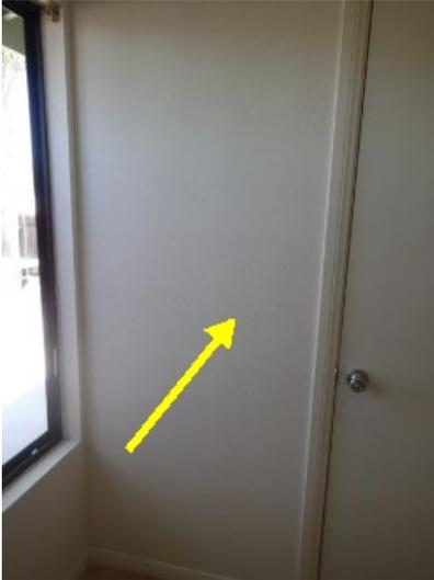
Sleeping areas are to have a switch at the door and either a outlet or ceiling light fixture controlled by that switch installed
