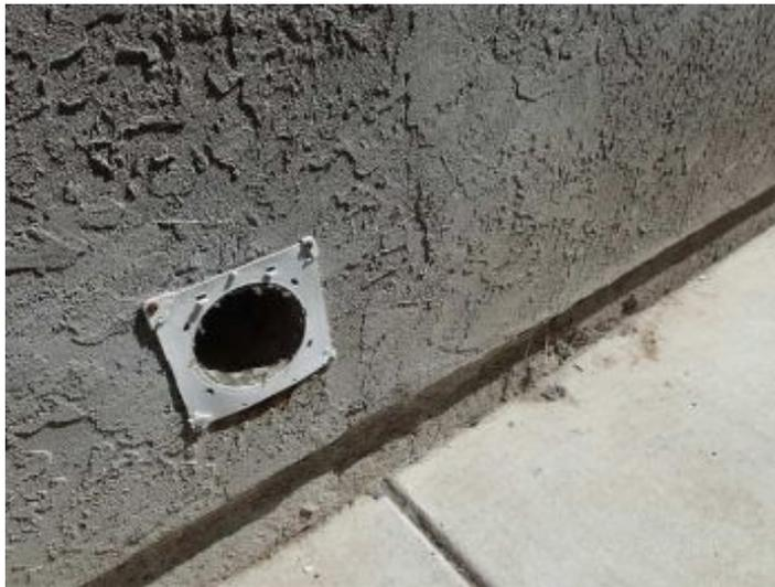
Vent rain cap and damper are missing on the outside of the building
