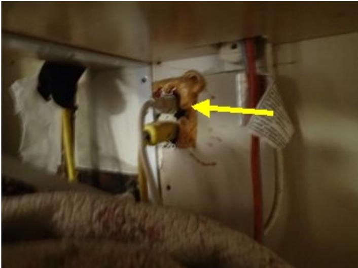
Some cover plates are missing from receptacles and switches. This situation can allow accidental contact of live electrical connections.
