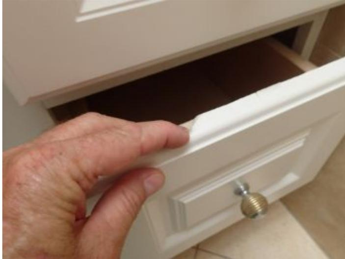
There is finish is degraded on the front of the cabinet drawer front top edge
